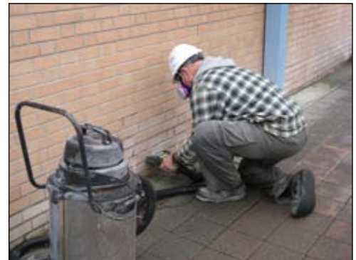
Tuckpoint grinding with LEV
