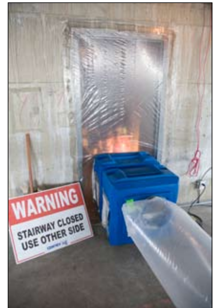
Poly enclosure with HEPA “negative air” unit
