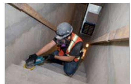
Stair grinding with LEV
