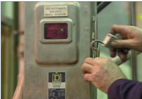
After disconnecting the machine from the electrical source, apply a personal lock.
