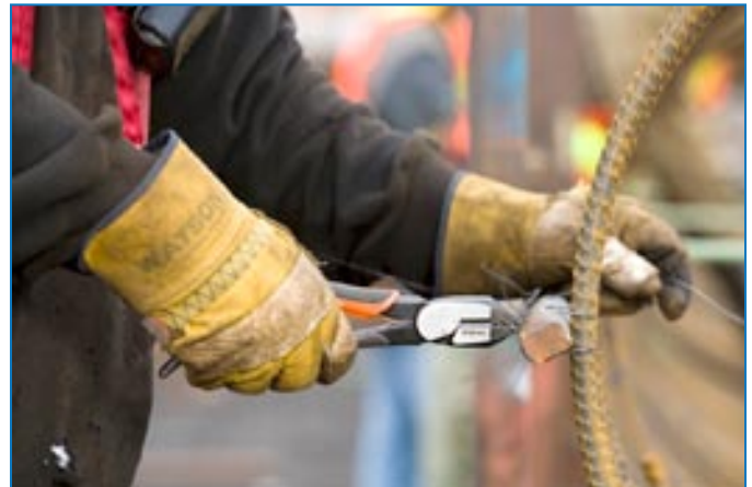
Wear gloves. An extra layer of fabric between the hand and the tool reduces pressure points on the palm.
